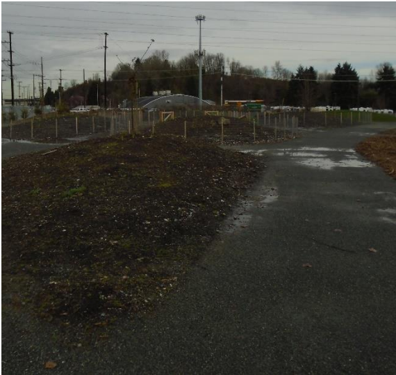
Figure 25: Approaching PH2-4 from the south on March 2, 2016
